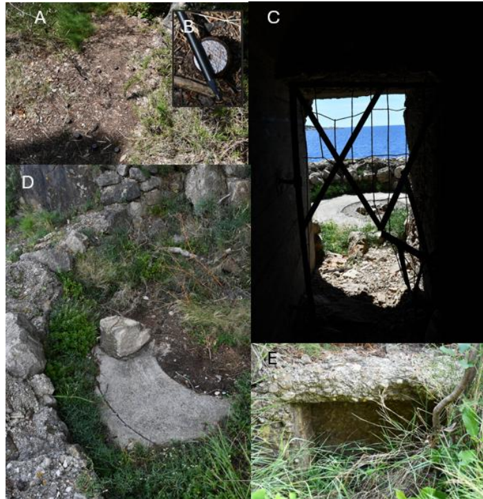
Figure 5: A: Bolts in concrete; B: Detail of a bolt; C: Tunnel entrance opening directly into a gun emplacement position; D: Concrete doughnut and surrounding parapet; E: Alcove in parapet.
