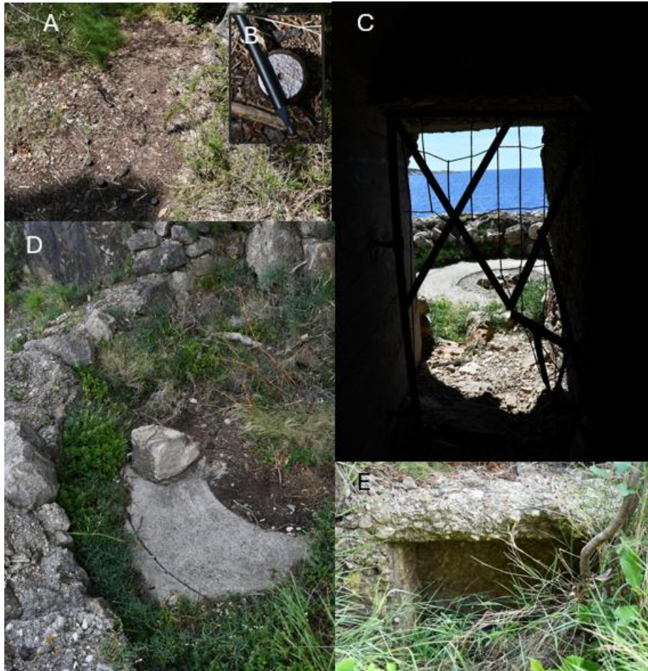
the base of a gun emplacement; B: Detail of a single bolt with pencil for scale; C: Tunnel entrance opening on to a gun emplacement; D: Surrounding parapet; E: Alcove in parapet.
