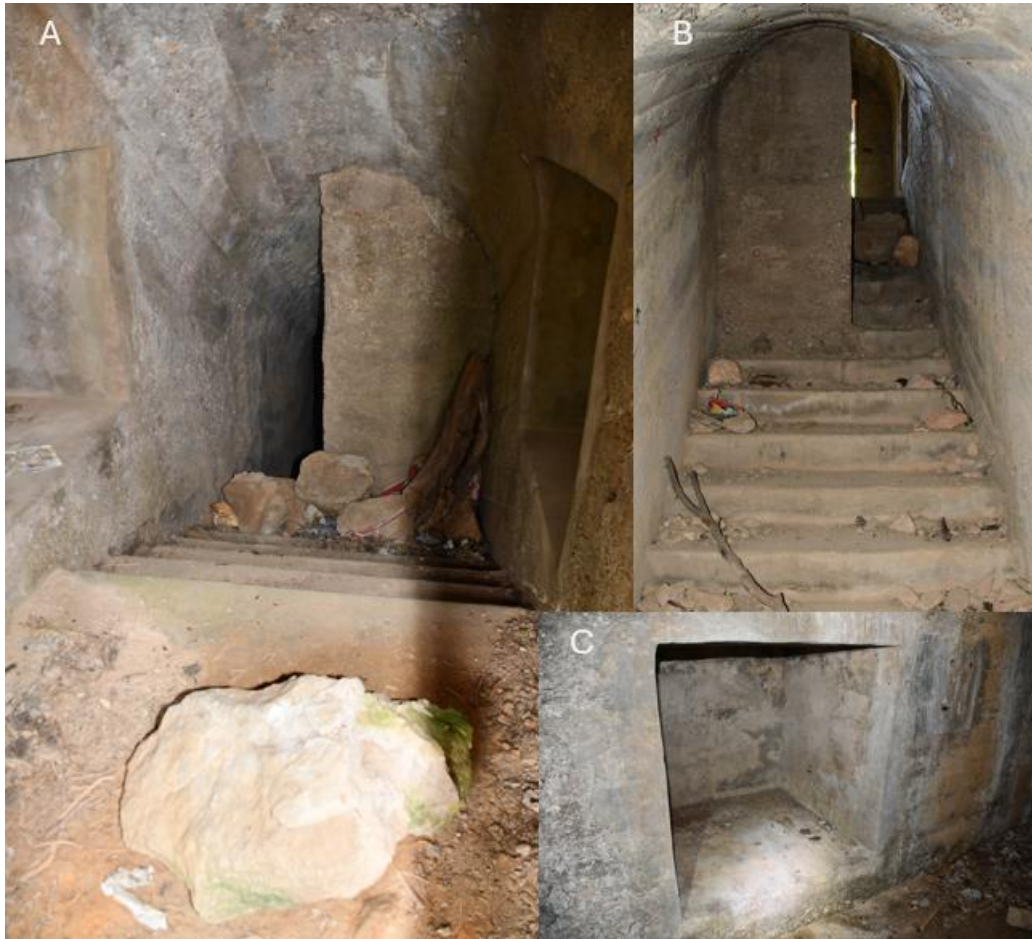
Figure 4: View looking into an upper-level gun emplacement entrance. Alcoves on the left and right and blast wall further back.
